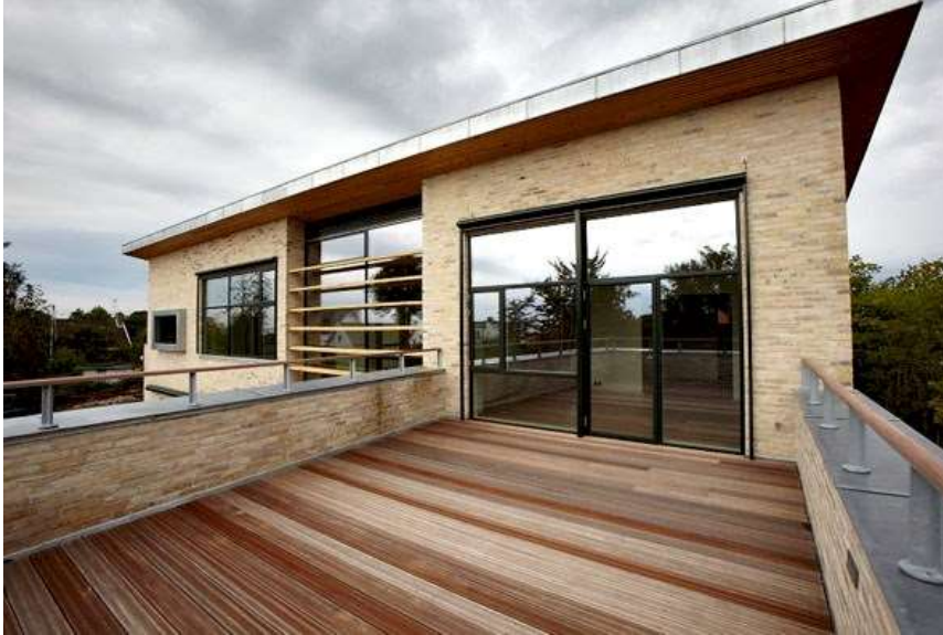
Figure 5. Use of reused bricks from Gamle Mursten in a modern villa, Denmark 15 .
