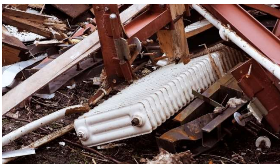
Figure 9. Various steel elements in the demolition waste.
