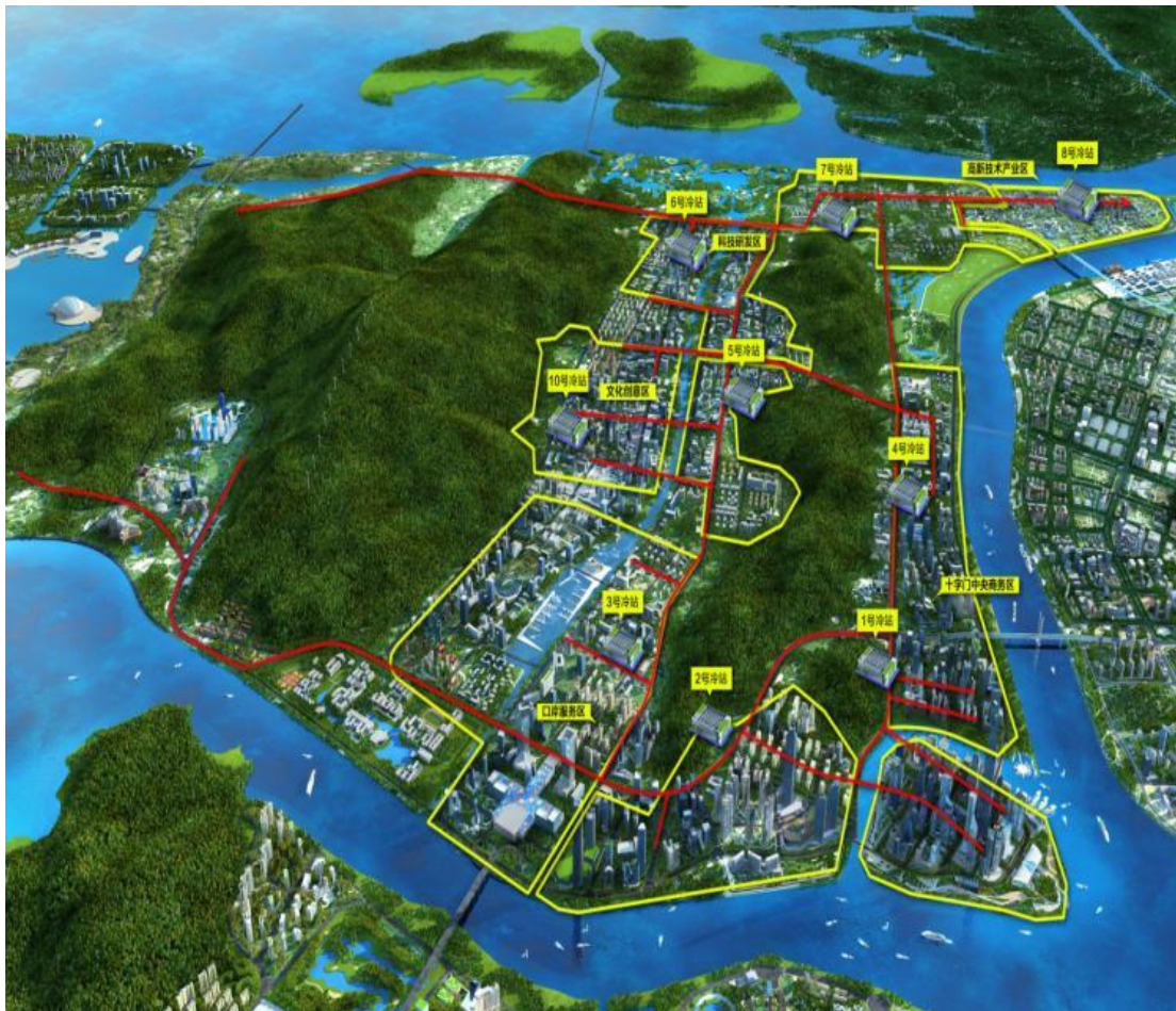
Figure 14: the DC system in Hengqin, PRC
