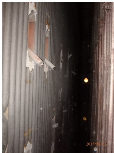
Figure 3. Commercial urea injection lances on the boiler front wall; secondary superheater on the right.
