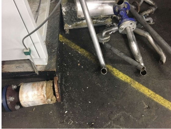
Figure 9. Oil spill (dark spots) on concrete floor in a machine hall. Photo: VTT
