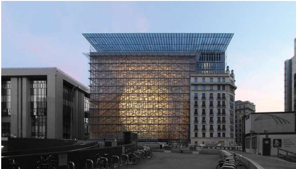
Figure 2. Façade of reused window frames in the Europa building, Brussels 9 .
