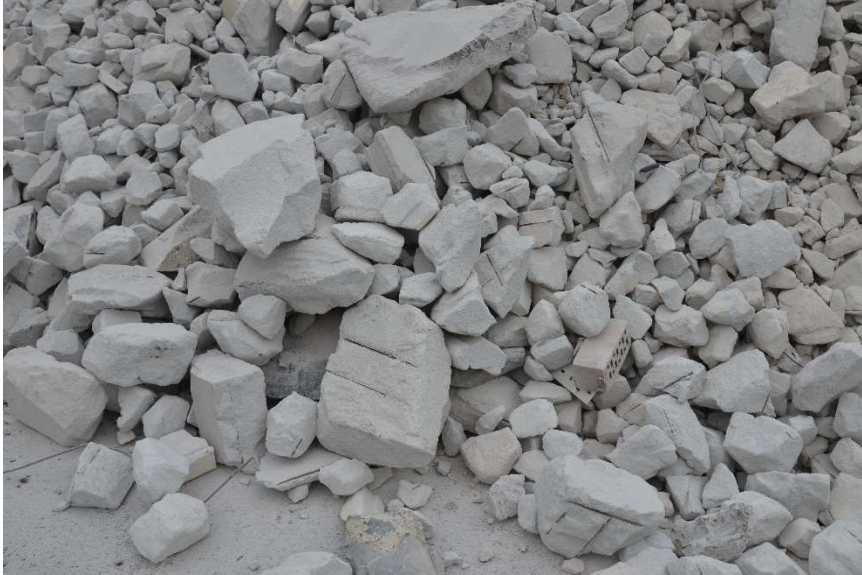
Figure 28. Separately collected AAC fraction during demolition works in Belgium, suitable for recycling in floor screed and cement stabilized sand.
