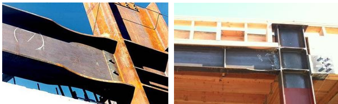
Figure 2. Application of Reduced Beam Section (RBS) Connection
