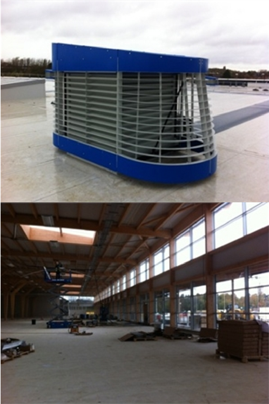
Figure 13: Windcatchers of a supermarket opened in January 2013 (courtesy of Monodraught Ltd).
