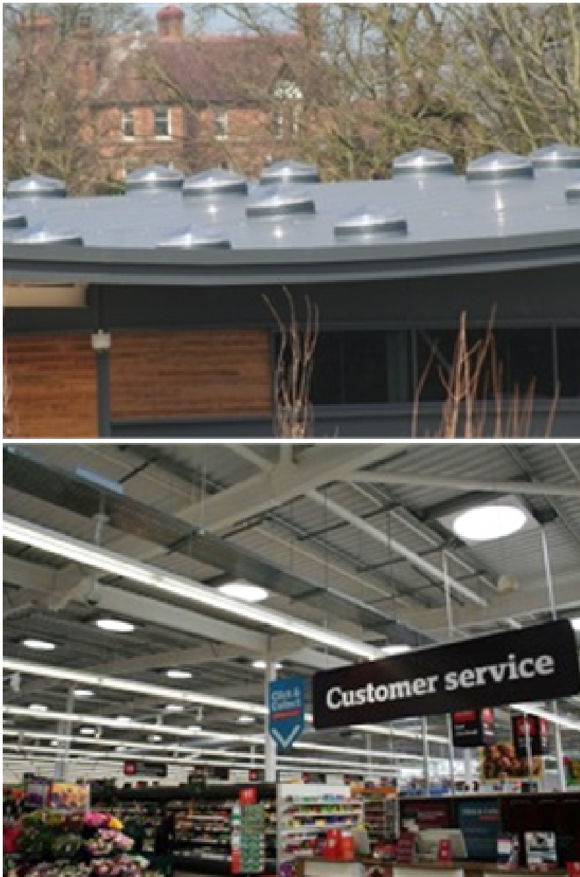
Figure 10: Roof lights of a supermarket opened in December 2012 (courtesy of Monodraught Ltd).
