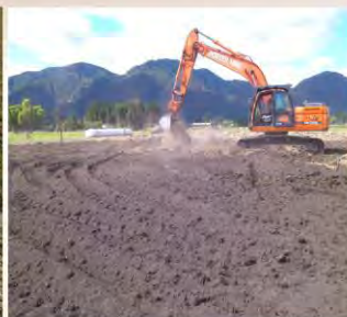
Fig 4. Excavating and mixing soil using a mechanised digger.
