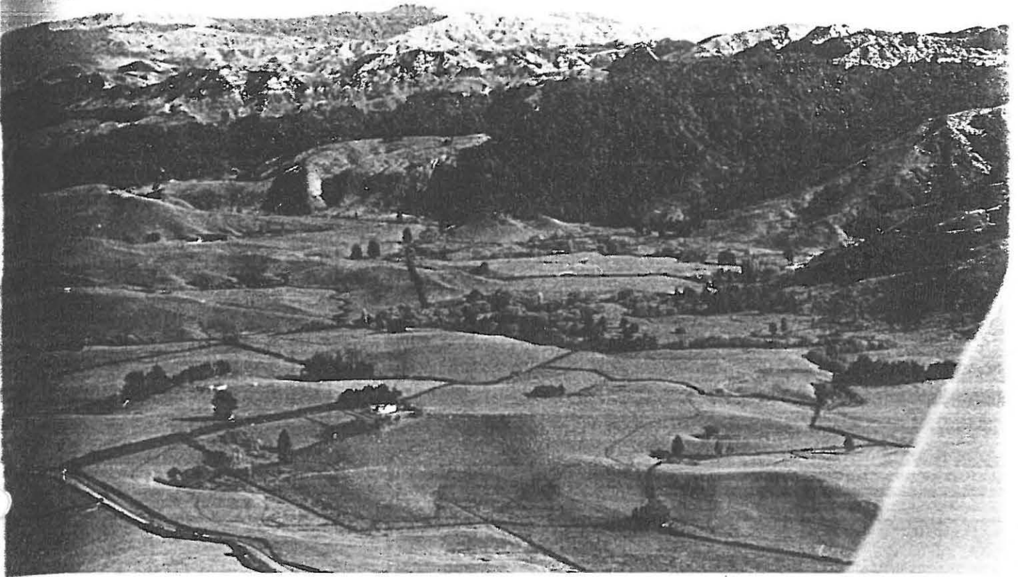
Figure 10.3 The western boundary of the Hamilton Basin near Whatawhata. The Waipa Fault Scarp forms a steep break between the undulating topography on early Quaternary sediments in the foreground and the higher greywacke hills capped by Tertiary sediments beyond. (MJ Selby)
