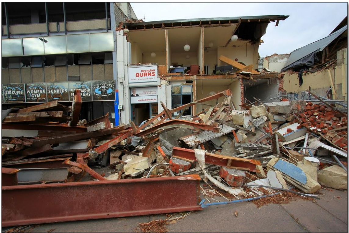
Figure 2.2: Damage to buildings in central Christchurch Source: BeckerFraser Photography 27 April 2011
