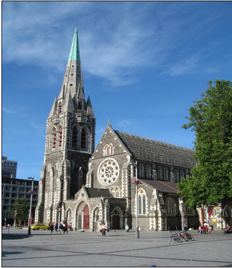
Figure 2.7: Christchurch Cathedral before earthquakes in 2010 Source: Greg O'Beirne, Creative Commons 20
