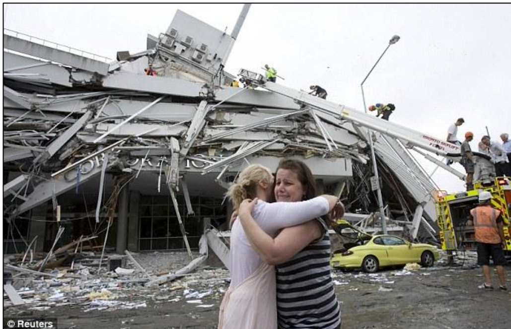
Figure 7.1: Collapsed Pyne-Gould Corporation Building which Chris saw out his work-place window (see page 132)
