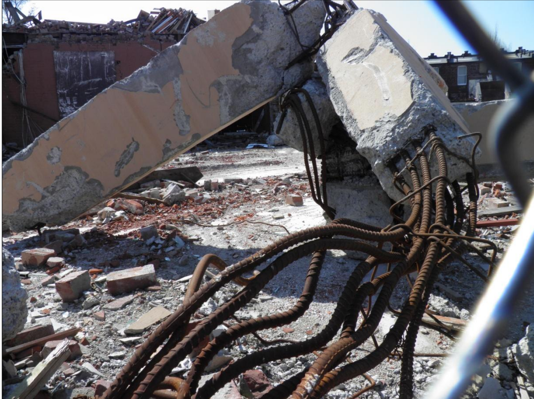
Figure 4.2: Through the CBD cordon: mangled remains of a trading store near the Cashel Mall Source: Author's own photograph
