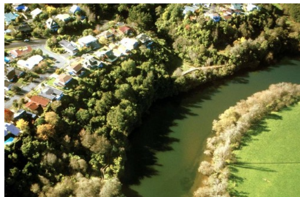
Figure 2. Hammond Bush, Waikato Riverbank, Hamilton. Adjacent is the mouth of a small gully system (part of the Mangaonua system), crossed by a 1.5m wide boardwalk. Indigenous evergreen vegetation (appearing as dark green) is clearly distinguished from the deciduous exotic vegetation (mainly Salix cinerea ).
