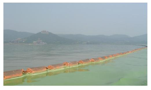
Figure 23 Outer wave-attenuation barrier installed to protect a water treatment plant intake in Lake Taihu, China (Photo: Liancong Luo)
