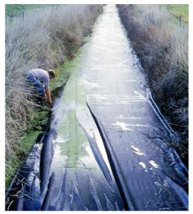
Figure 13 Surface cover fitted over a ditch system to control aquatic vegetation (Photo: R. Wells, NIWA).
