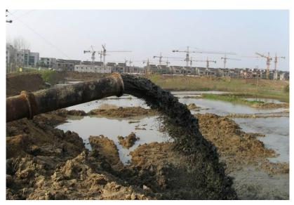
Figure 21 Dredged spoil pumped from a dredging operation on a lake on the Yangtze River delta (China).
