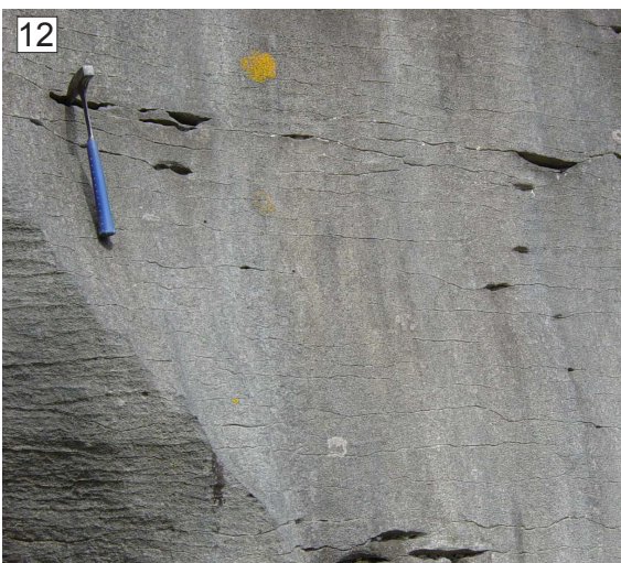
Fig. 13C Field photos of locations at C50 identified on Fig. 13A.
