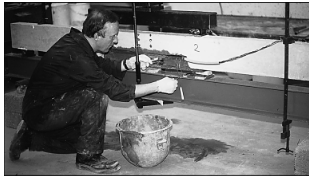
Fig. 2. Application of hand-applied repair, unpropped beam
