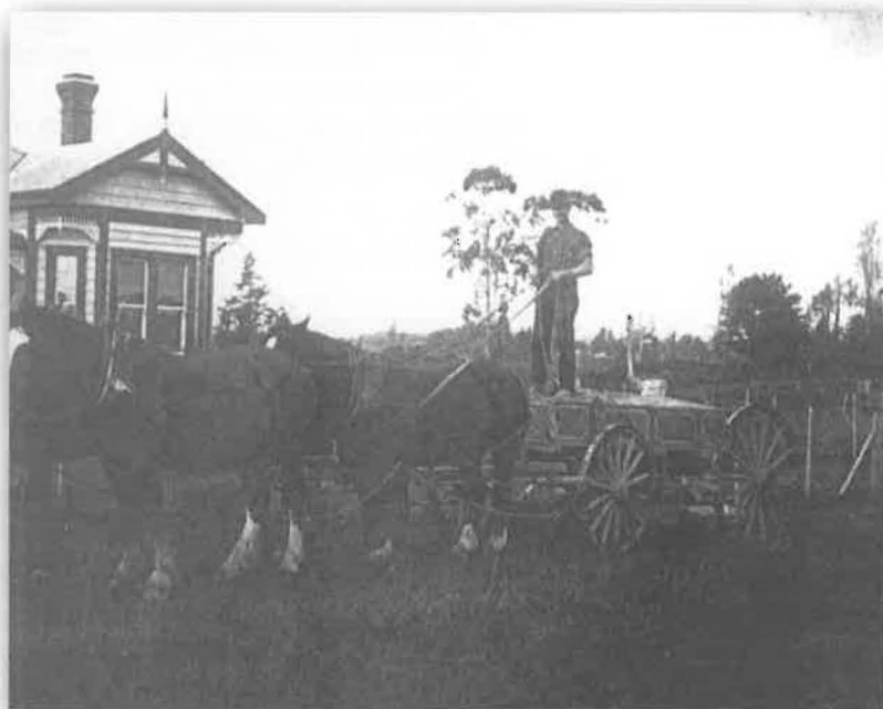
FIG 3.2 Mr G Reynolds outside Mr W Melville's house on the corner of Mangapiko Street, Te Awamutu with his team of horses and load of sand for Tokanui buildings. In the years 1910 – 1912 Mr George Reynolds with his team of horses carted the metal and timber and sand to Tokanui to build the Superintendent's house and the hospital. The first of the hospital buildings was finished and the patients moved to their new home in July 1912.
