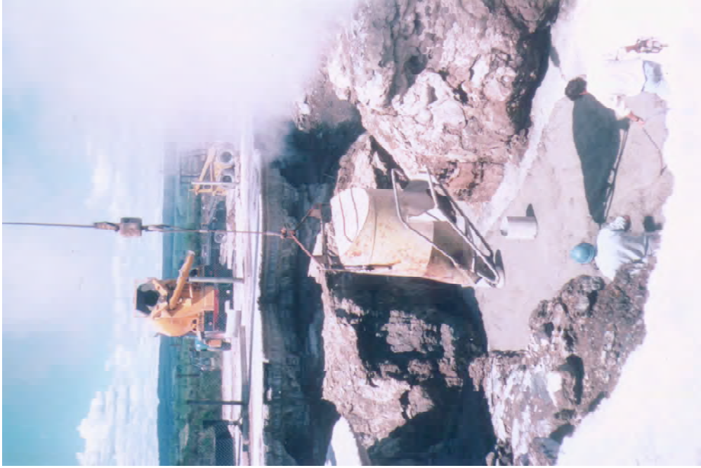
Ohaaki Pool: top left , the Ngawha filled with water and some rejuvenation of collapsed sinter formations, November, 1988, before power station commissioned; bottom left , the Ngawha drained in June 1989; right , grouting the floor of the Ngawha, October 1989.
