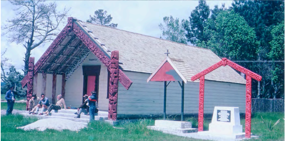
Restoration of Te Ohaaki Marae: top . November 1981, land around the marae has been cleared; middle . May 1982, the meeting house has been raised and reblocked with a new concrete porch and steps, and a new roof put on; bottom . November 1982, the carvings have had conservation work done and put back on the meeting house.
