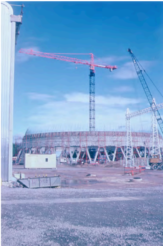
Construction of the cooling tower, Ohaaki power project: top left , the hole for the foundation, August 1985; bottom left , building up the rings of concrete, July 1986; right , the tower takes shape, May 1987.
