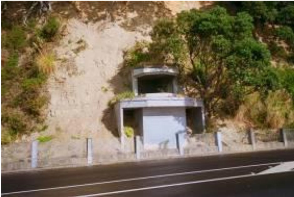
Figure 7. Photograph of Brett's "cave" (a gun emplacement)
