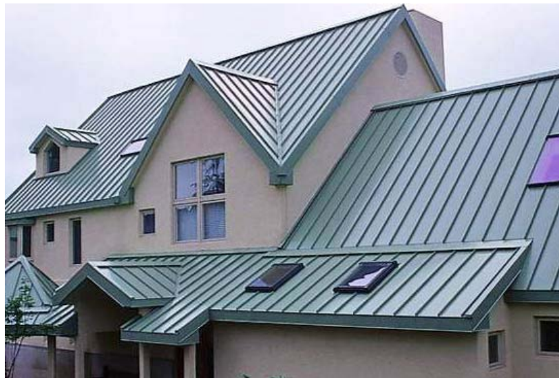
Fig. 1 Long Run Metal Roof
