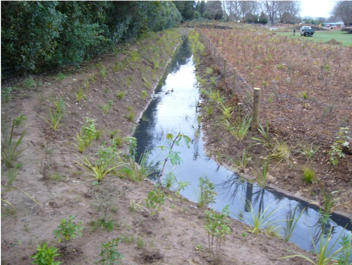
Plate 2: Newly installed drain along the western boundary, created in 2009
