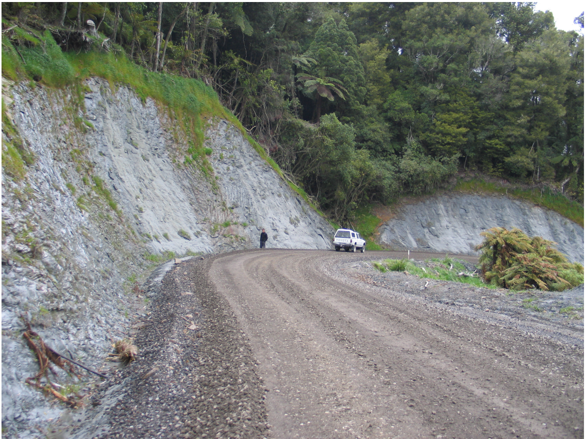
Fig. 43: Photo of section on the Tongaporutu-Ohura Road, east of Kotare Stream, showing the lower part of Otunui Formation. Stop 17, R18 – 661 597.
