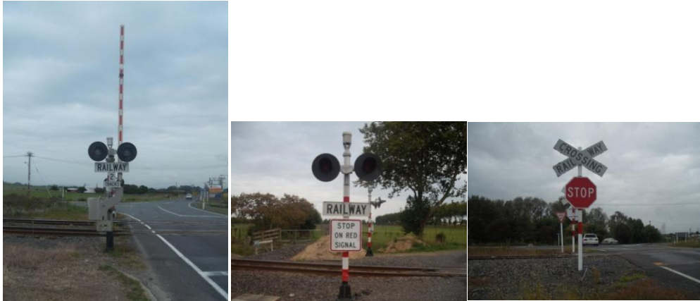
Figure 2: Photos of the warning protection devices used in New Zealand. From left - Active protection system with half-arm barrier, active protection with warning bells only, passive protection system.
