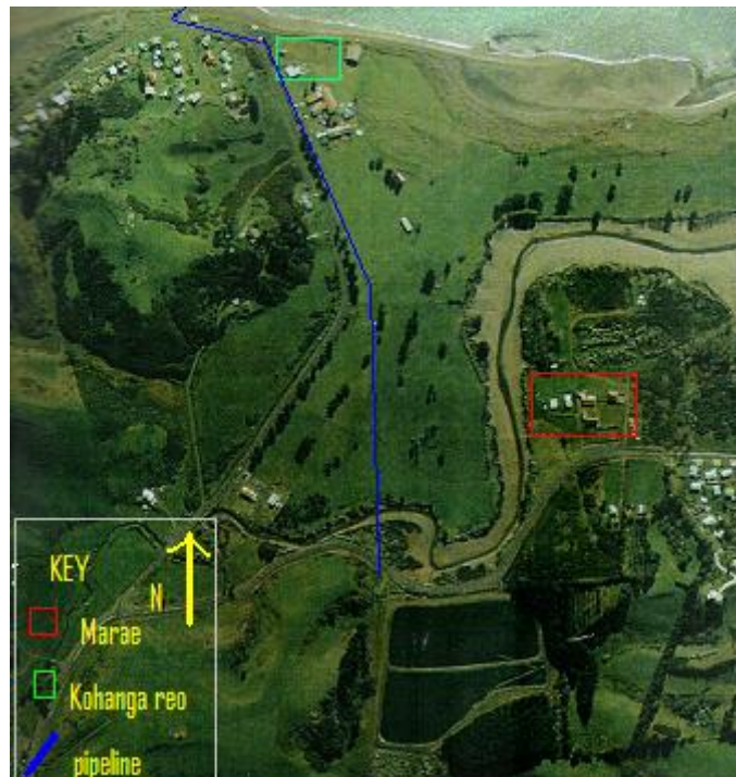
Figure 8: Pipeline illegally embedded in Tainui land
