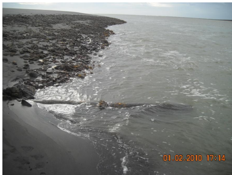
Figure 7: Sewage discharge pipeline entering the moana at te Kopua.
