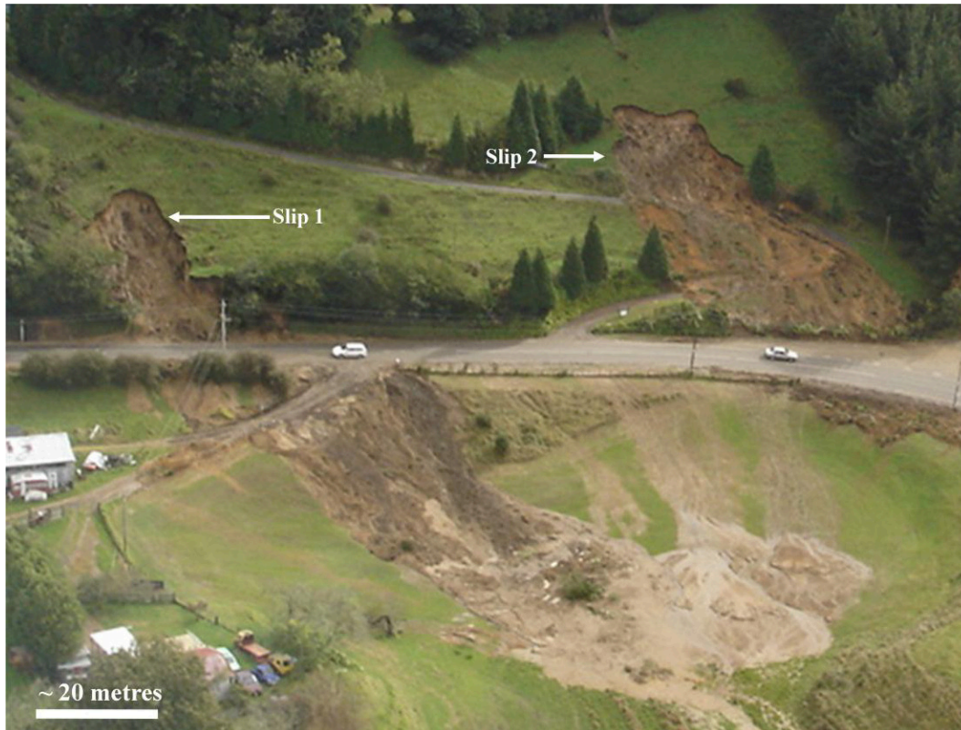
Figure 4.3: Slips on Welcome Bay Road at Welcome Bay. Note the distinction between slip 1 and slip 2 and the run out distances of each slip (Photo courtesy of Tauranga City Council).
