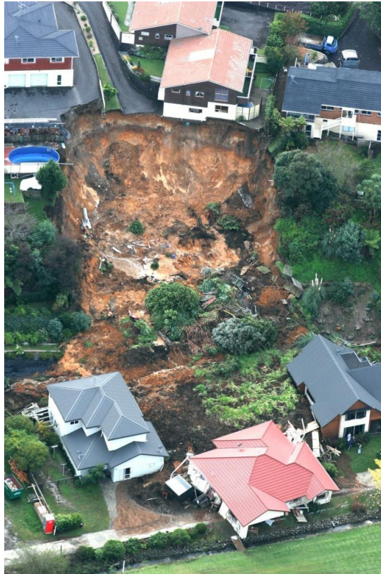
Figure 2.4: Slip at Vale Road, Otumoetai. Note little debris remains in the scarp and the house with the red roof has been pushed off its foundations (Photo courtesy of Tauranga City Council).
