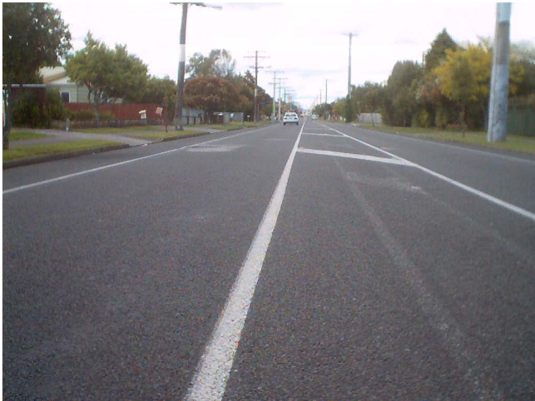
Figure 3: Road to be redesigned in the workshop (North facing).
