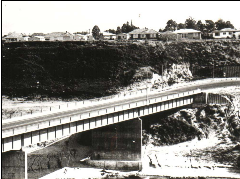
Figure 4.2 Cobham Bridge shortly after completion. It serves as a crossing for State Highway 1 which runs through the city. See Appendix A.1 for location.
