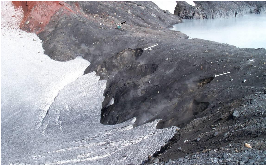
Fig. 2.10 Seeps and erosion of the tephra dam face caused by piping by February 2007. White arrows indicate seeps #4 and #6 (left to right) that were the locations of initial failure. The black arrow indicates a GNS scientist and equipment station for scale (GNS photo archive).
