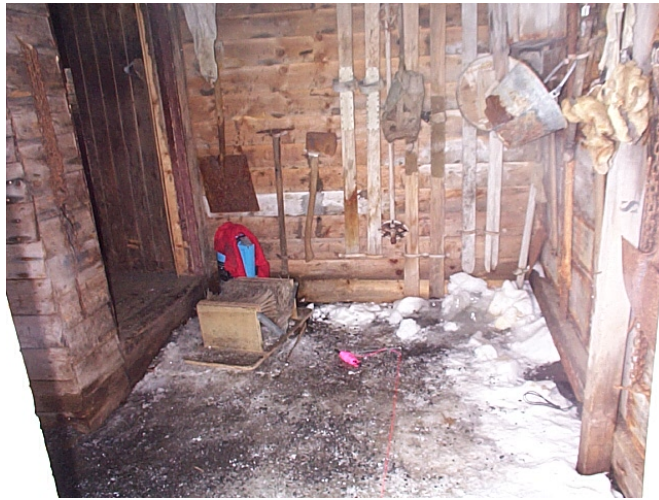
Figure 1.20: Photograph of the annex area with the main door to the hut on the left (Source Professor Roberta Farrell, 2002).
