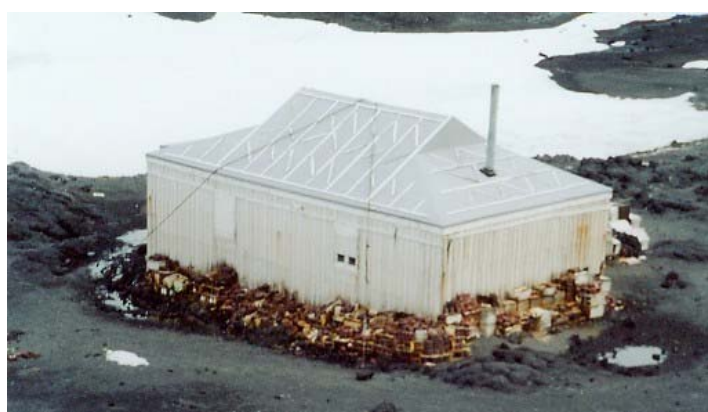
Figure 3.23: Photograph of stores around southern and eastern side of the Nimrod Hut. (Source, Professor Robert Blanchette 1998).
