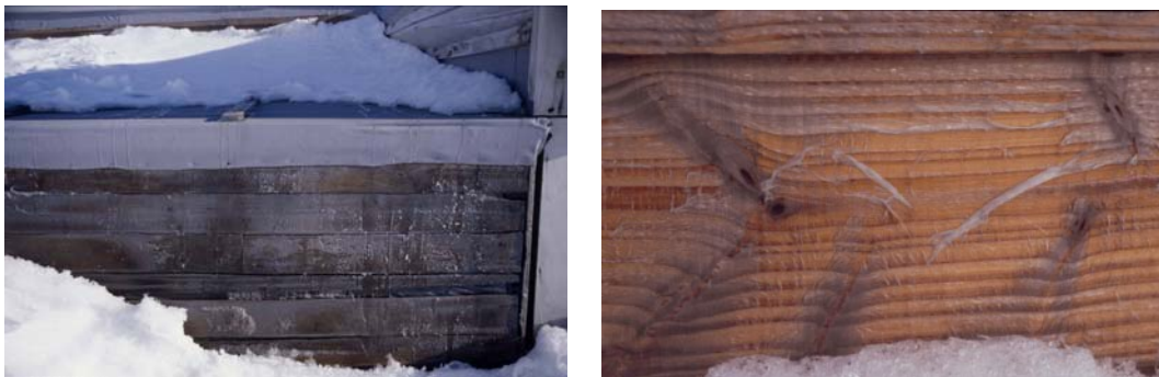
Figure 2.1: Photographs of wood defibration Left: Stable wall Terra Nova hut showing ice melting down the wall. Right: Closer photograph showing layers of wood cells washing off in the melting snow (Source Professor Robert A. Blanchette, 1998).
