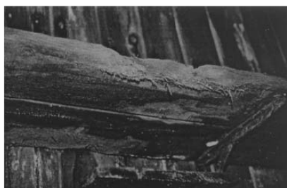
Fig. 7. Chemical spill inside the Cape Evans hut causing a deterioration of the wood. High concentrations of chromium and lead are associated with this caustic chemical spill.
