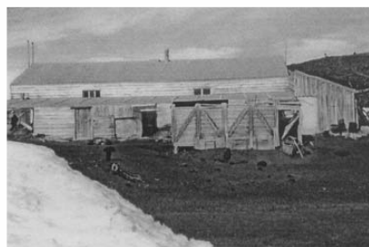
Fig. 5. Snow-free area round Cape Evans hut that contains several hundred pieces of asbestos on the surface of the ground.
