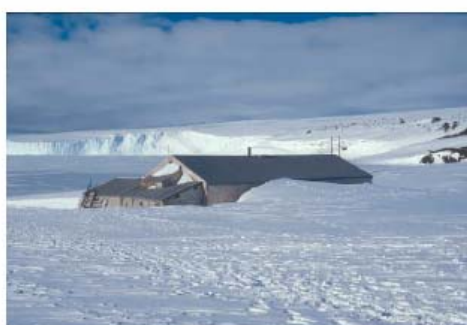
Fig. 5. Cape Evans hut in mid December showing a large amount of drifting snow that accumulates over the winter months.
