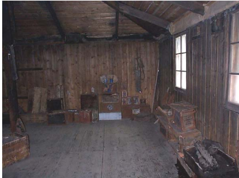
Figure 1.15: Photograph inside the main area of Discovery Hut (Source Professor Robert A. Blanchette, 1998).
