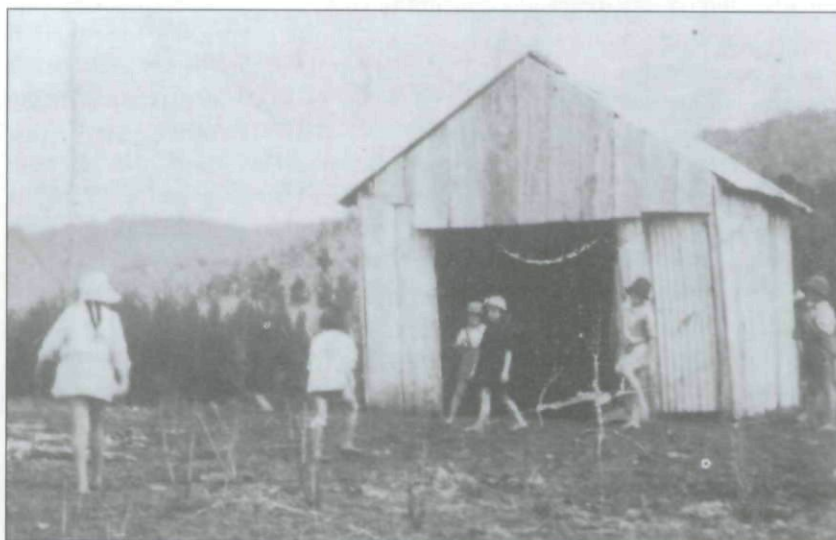
Figure 1: Kohua Road School in 1927 provides a good example of the sub-standard state of some small schools in the 1920s. 35
