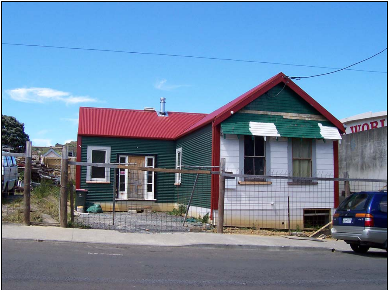
The former Wigan St cottage on its new site in Newtown where implementation of the consent for the additions and alterations is nearing completion. It is recommended that this building be removed from the heritage list as a result of the consented activities. Photo by Ann McEwan on 01.12.2004.
