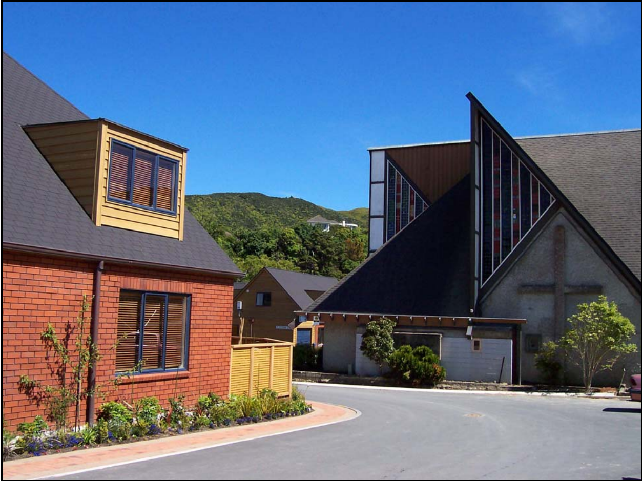
Contrasting designs - a completed unit on the Friend St boundary. Photo by Ann McEwan on 30.11.2004.
