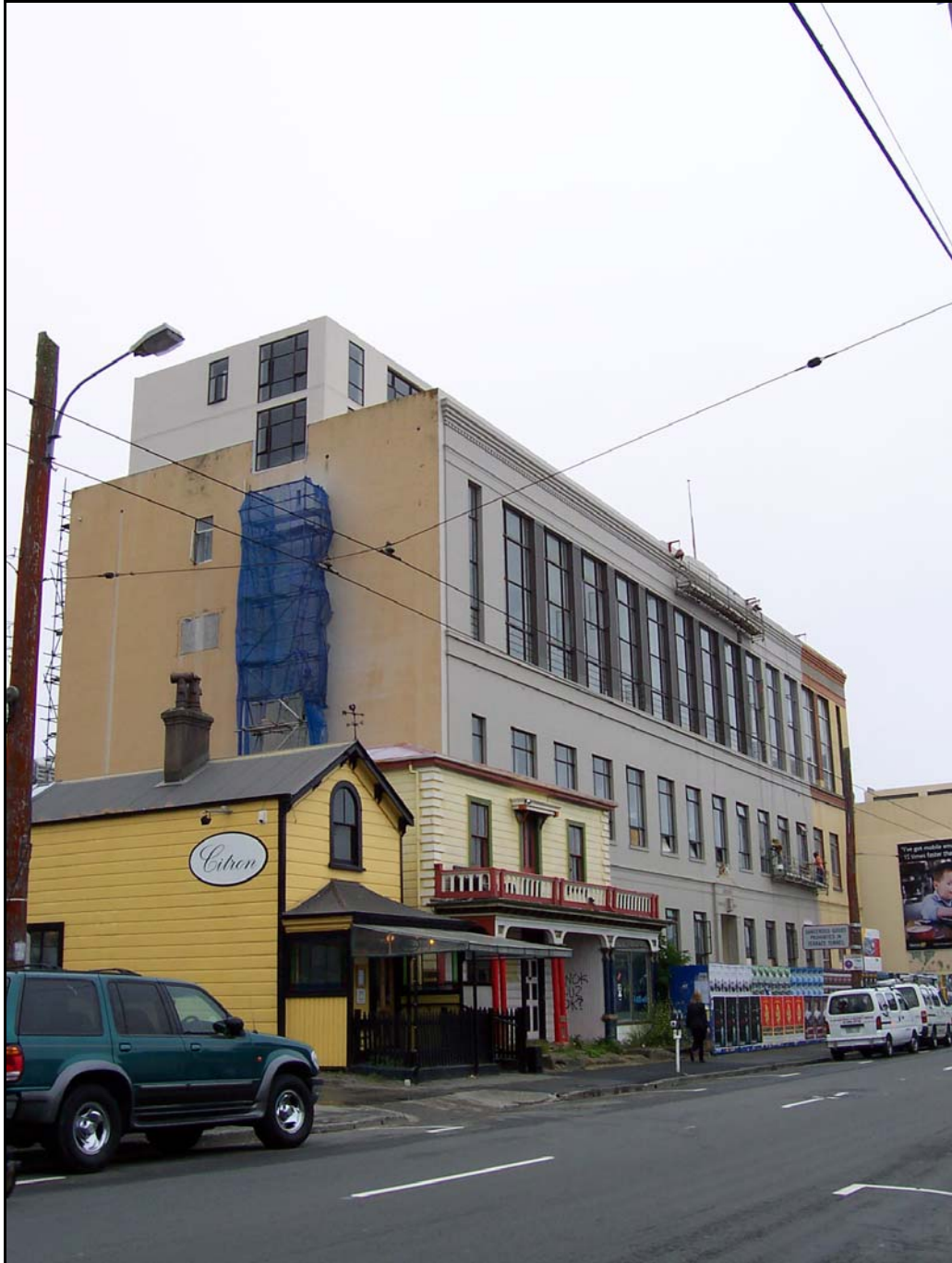
View of the listed building and the rooftop addition looking north up Willis St. Photo taken by Ann McEwan on 02.12.2004.
