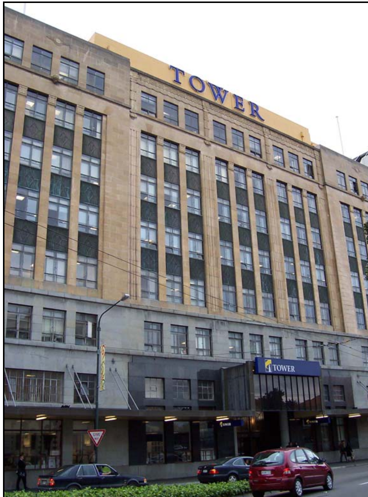
Government Life Building with new 'Tower' signage on upper Customhouse Quay facade. Note the canopy proposed to be replaced by SR 33493 is still in-situ. Photo by Ann McEwan, 10.11.2004.
