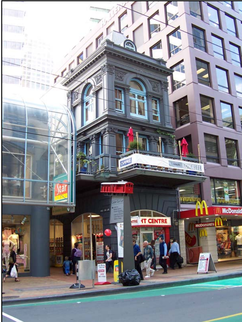
Kelburn Chambers from Lambton Quay showing the new balcony and associated work undertaken under SR 57761. Photo by Ann McEwan on 03.12.2004.
