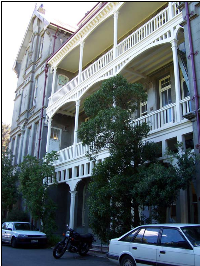
A view of the restored verandah on the front of the Erskine College Main Block Photo by Ann McEwan, 01.12.2004.
