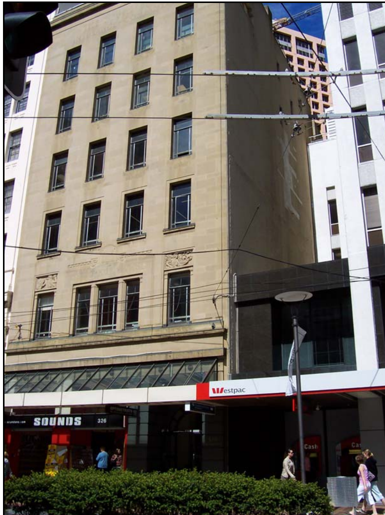
View of the South British Insurance Building from Lambton Quay – note the removal of building identifiers from above the 1 st floor windows and at parapet level. Photo by Ann McEwan on 03.12.2004
