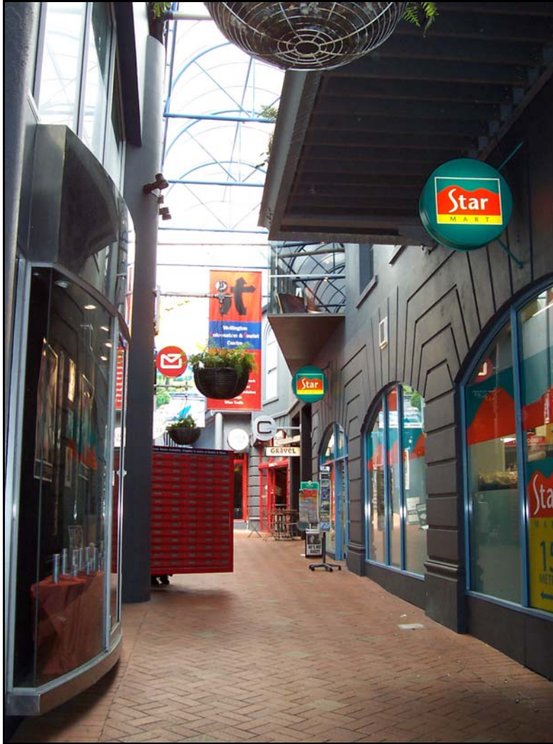
View down Cable Car Lane showing the 1 st floor window protrusion (SR 48429) and the recent Star Mart (SR 75930). Photo by Ann McEwan on 03.12.2004.
