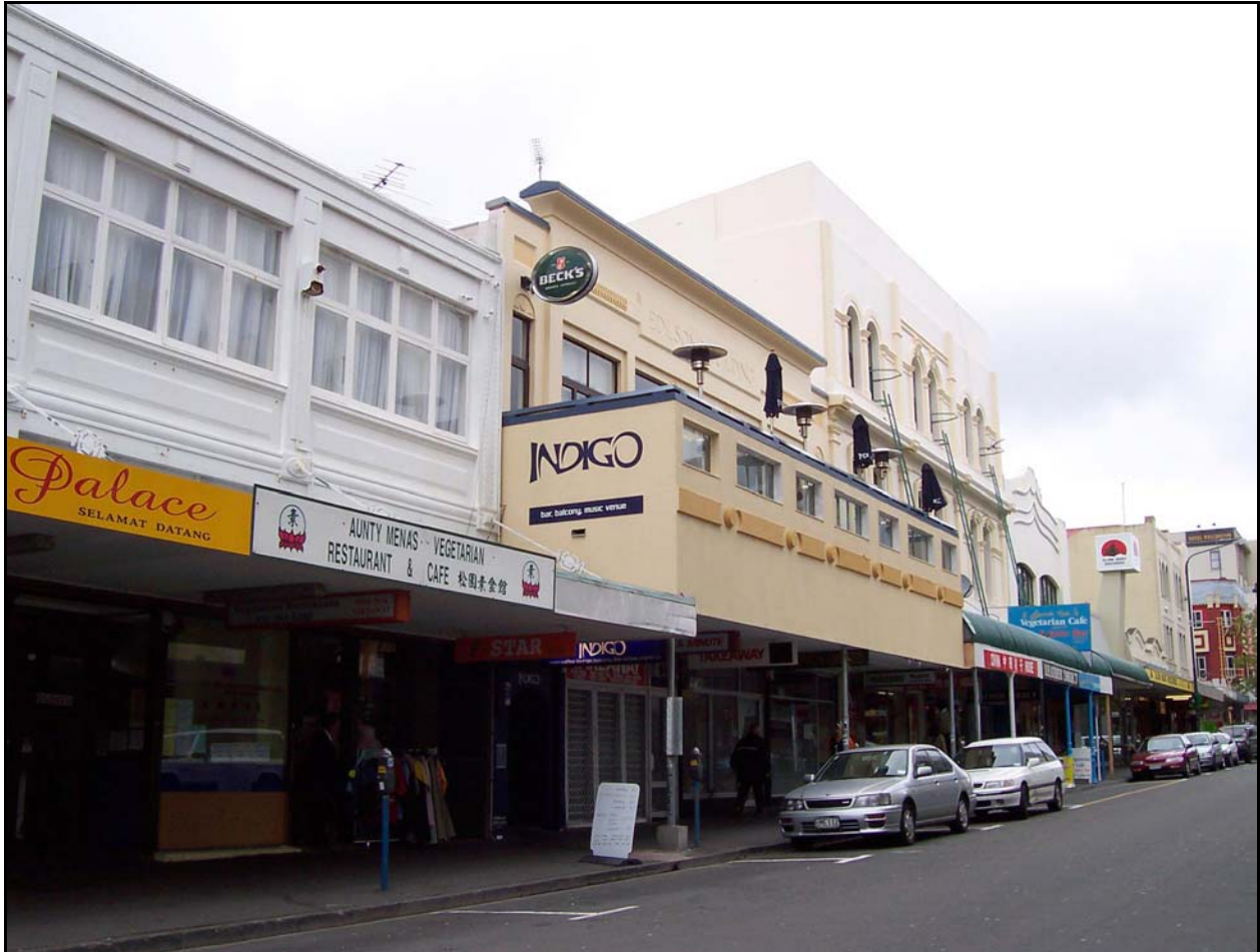
The Johnson & Edilson Building after the balcony (SR 81024) was erected. Photo by Ann McEwan, 09.11.2004.
