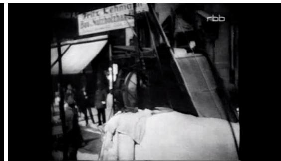
Figure 3.1.14 A shot from the front of the tram (backwards)
