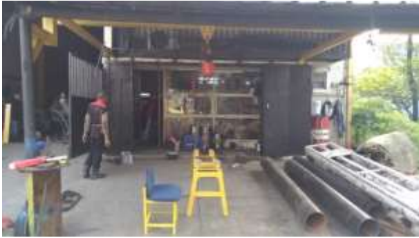
Figure 8. The workstation of Pipe Welding
