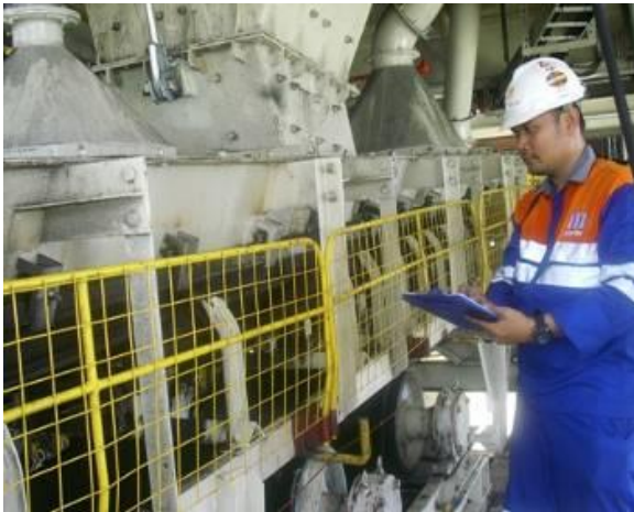
Figure 4. Assessment of coal handling facility by consultant
