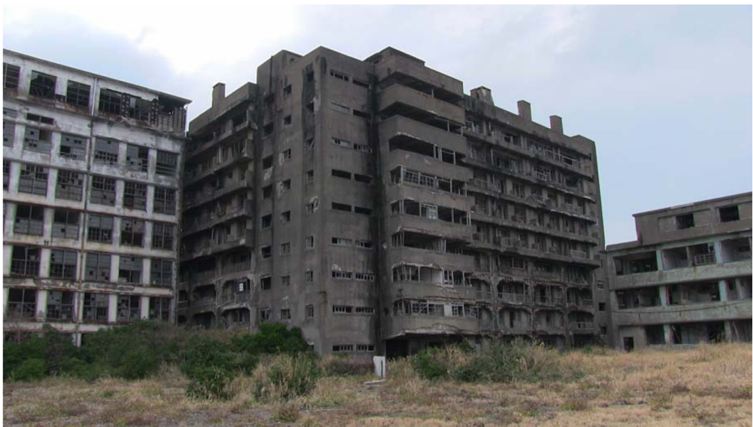
Figure 2. [In color online.] Apartment building (photograph by Peter Matanle, ©Peter Matanle).
