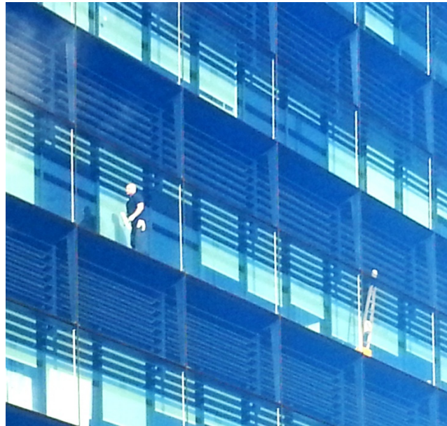
Figure 12. Blinds in drawn position, South façade, Kings Place, London, Dixon Jones.
