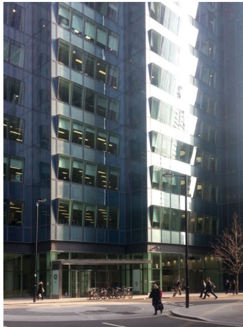
Figure 3. South facing inclined windows, Ropemaker Place, London, Arup Associates.
