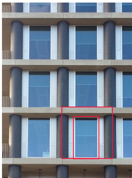
Figure 6. Typical façade detail showing glazing percentage. One Pancras Square, London, David Chipperfield Architects.
