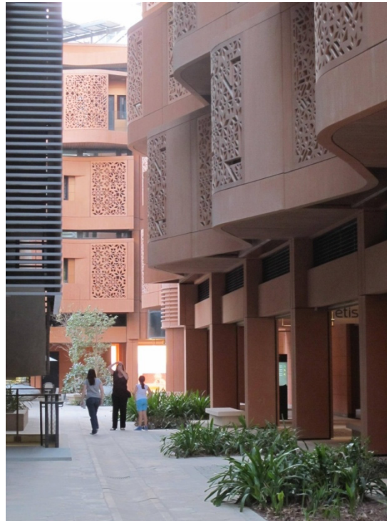
Figure 1. Shading by adjoining building, façade modelling and limited glazed openings, Masdar, Abu Dhabi, Foster and Partners.
