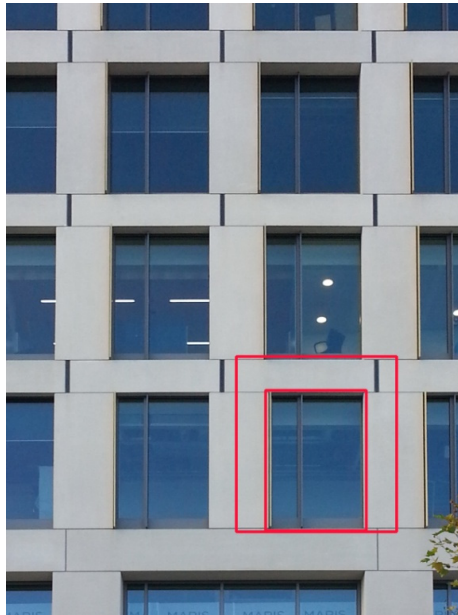
Figure 8. Typical façade detail showing glazing percentage. Two Pancras Square, London, Allies and Morrison.
