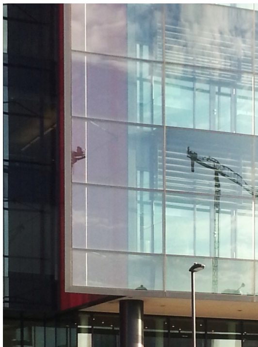
Figure 10. Close-up of double skin façade, Kings Place, London, Dixon Jones.
