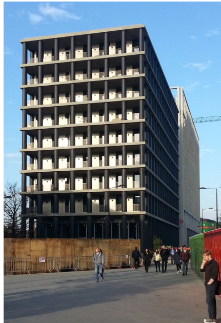
Figure 5. South facing portico with cast iron columns. One Pancras Square, London, David Chipperfield Architects.
