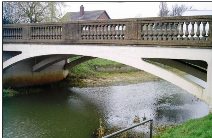
Plate 12.2: The SF2 (Donington Bridge) survey site (OSGR: TF-17300-35600). Glyceria maxima (Hartm.) Holmberg was the dominant vegetation at the SF2 (Donington Bridge) survey site. (Photograph taken 30th March, 2010)
