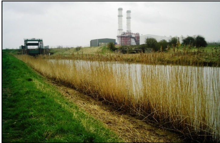
Plate 12.8: The SH4 (Nene Outfall Sluice) survey site (OSGR: TF-47400-19900). The sluice can be seen in the background, as can a power station. Phragmites australis (Cav.) Trin. ex Steud. can be seen extending along the banks of the South Holland Main Drain. (Photograph taken 29th March, 2010)
