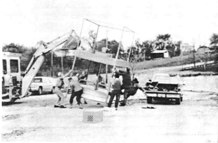
Figure 1. Completely assembled aerator prior to its installation
