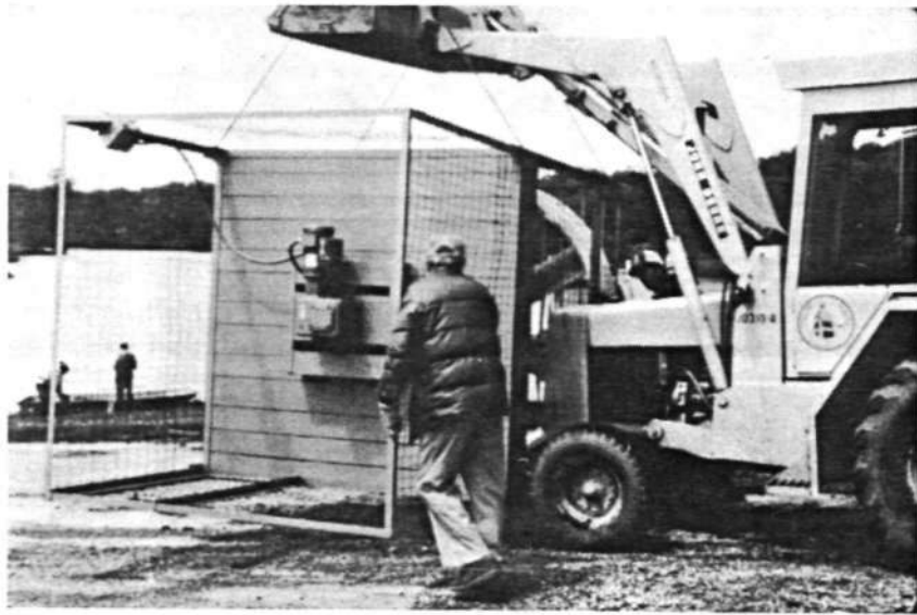
Figure 3. View of the platform, motor, and reduction gear
