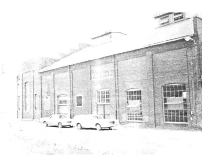
Figure 4. Main building of water plant at Alton
