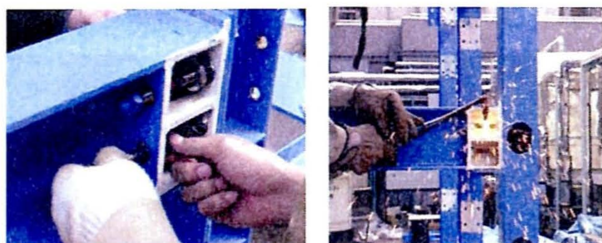
(c) 鋼棒の切除(逆回し)
