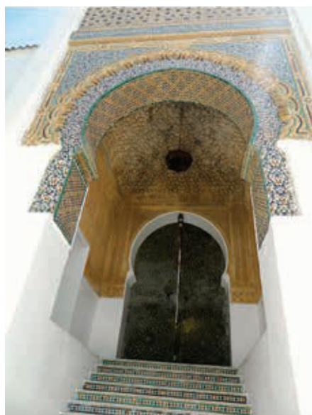
Figure 3. The front porch with a triple festoon of bricks inlaid with an enameled green netting pattern. Source: Authors.
