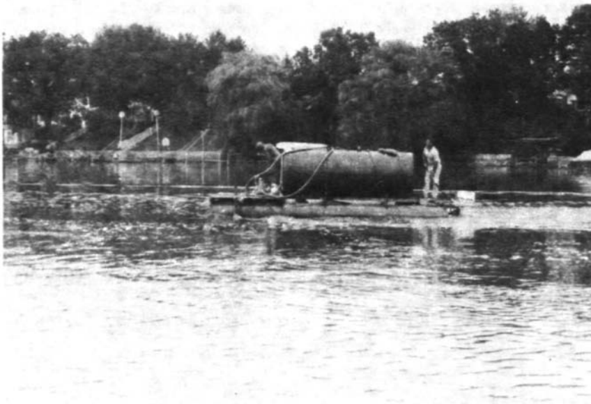
Figure 6. View of the pontoon tank fully loaded
