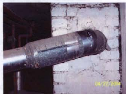
Figure 10 - Gap in furnace flue
