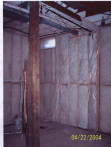
Figure 2 - Vapor barriers on the basement studs
