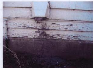
Figure 5 - Clogged dryer vent.
