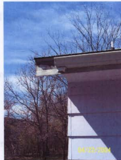
Figure 2 - Missing downspout.
