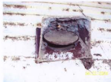
Figure 3 - Dryer vent port in open position.
