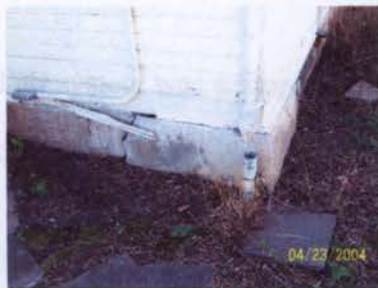
Figure 4 - Cracked foundation
