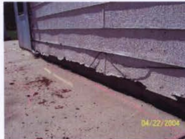
Figure 3 - Damaged siding.
