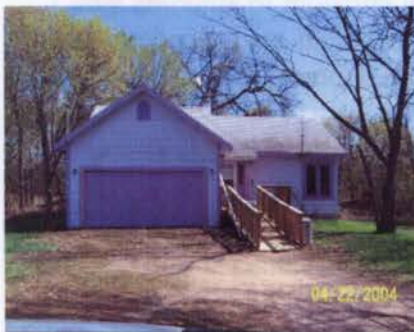
Figure 5 - Home with good site drainage
