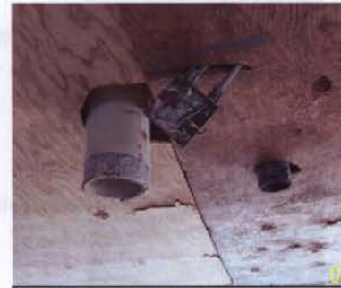
Figure 9: Penetrations through platform
