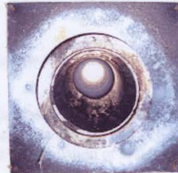
Figure 8: Looking up through abandoned stove pipe
