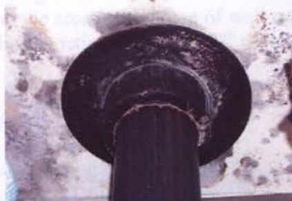
Figure 6: Stove pipe at ceiling
