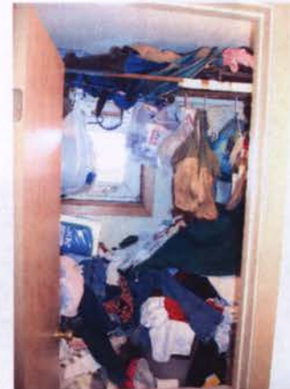
Figure 2: Clutter causes condensation problems on exterior walls.
