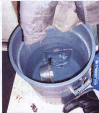
Figure 7: Bucket with water in hallway
