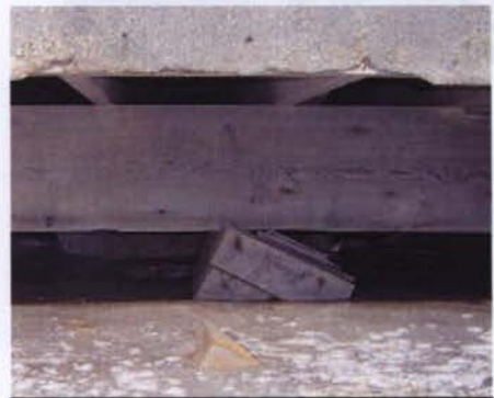
Figure 7: Pier, support beam and floor joists
