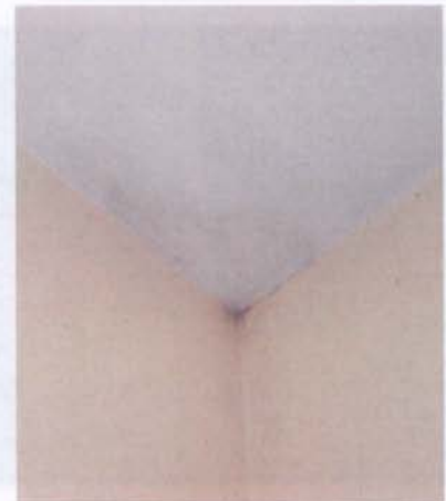
Figure 4 - Upper level wall/ceiling junction
