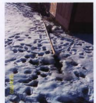
Figure 3 - Sump Pump Discharge
