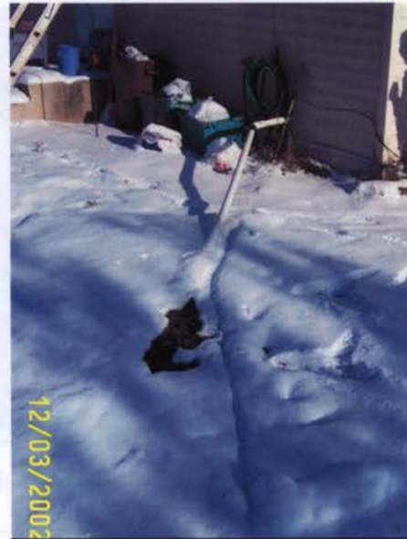
Figure 4: Outfall from basement sump pump.
