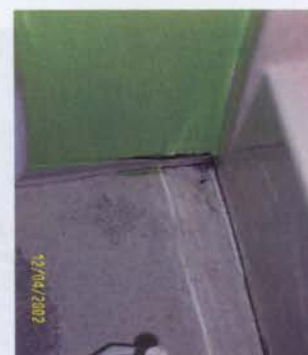
Figure 2 - Mold at Bathtub
