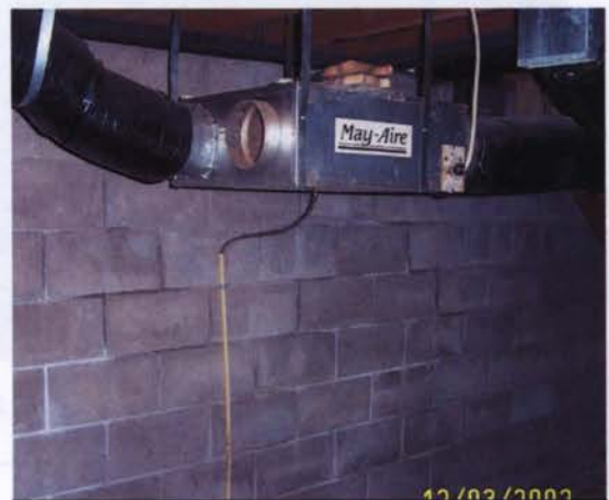
Figure 5: Heat Recovery Ventilation System
