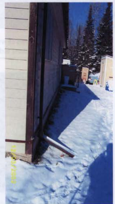
Figure 2: Downspout and leader at rear of house
