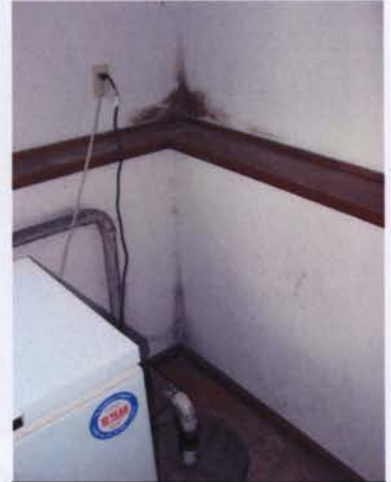
Figure 1 - Lower level, exterior corner @ sump
