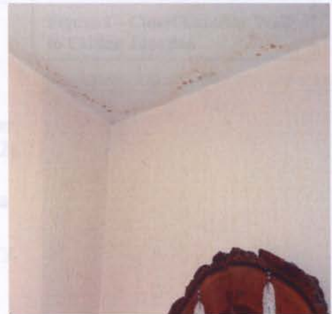
Figure 5 - Water Stains
