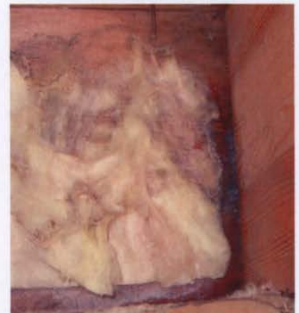
Figure 3 - Frost on Band Joist
