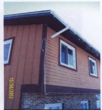
Figure 1 - Broken Downspout
