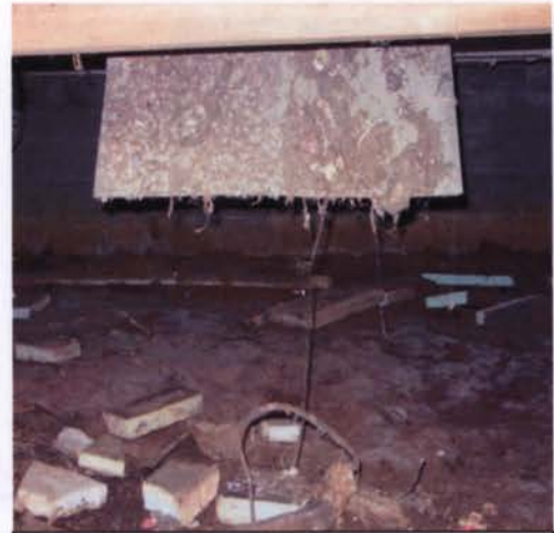
Figure 4 - Open Return Air Plenum
