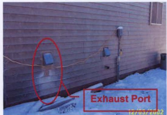
Figure 6: Exterior ports for HRV system
