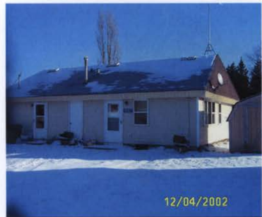
Figure 1 – 58817 Circle Drive Front Elevation
