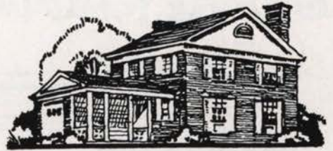
The I=B=R Research Home at the University of Illinois where research in steam and hot-water heating is conducted.
