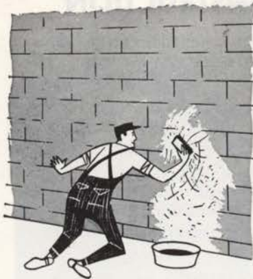
Scrub cement base waterproofing into basement wall to eliminate seepage.
