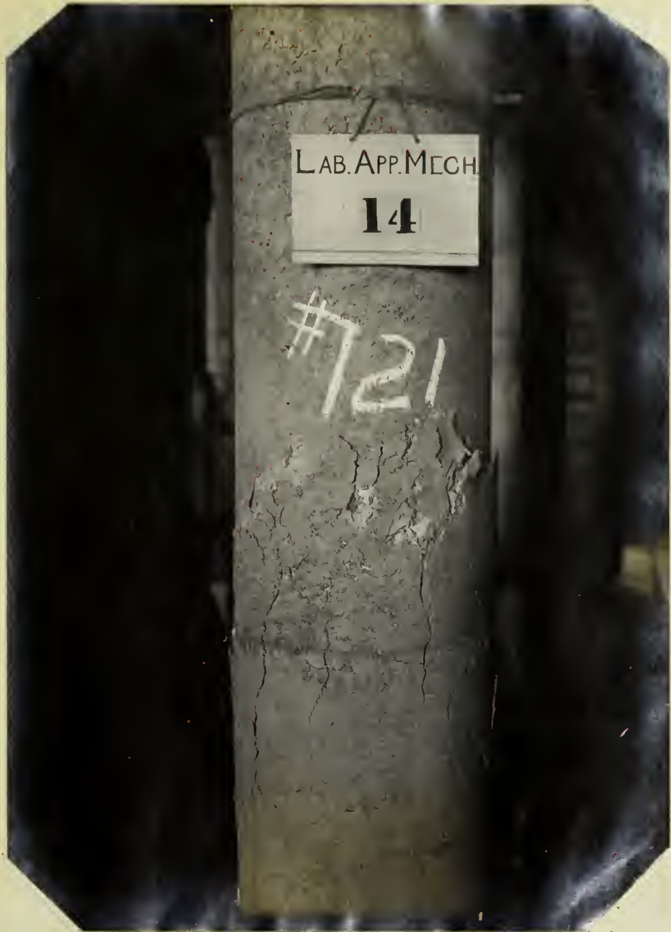
View Showing Typical Crushing Failure. This Column was tested in the 1907 series.
