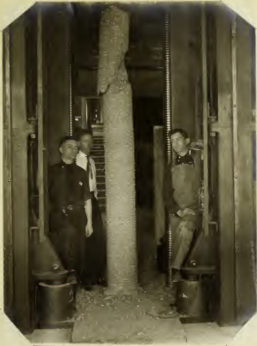
View showing Spalling failure in column after being stripped of Reinforcement.
