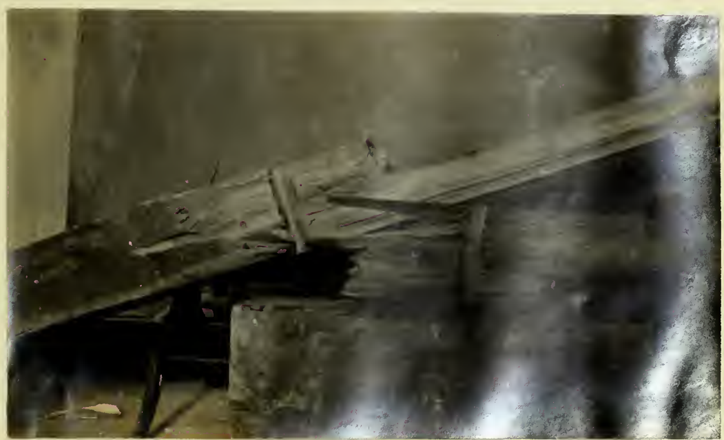
E 3. Showing character of failure.
