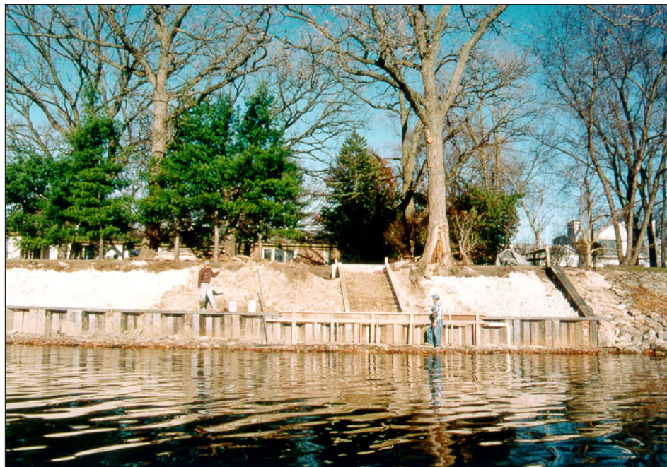
Figure 7b. An example of the installation of bank protection residential sheet-piling on the Kankakee River in Kankakee, Illinois (from Bhowmik and Demissie, 2000)
