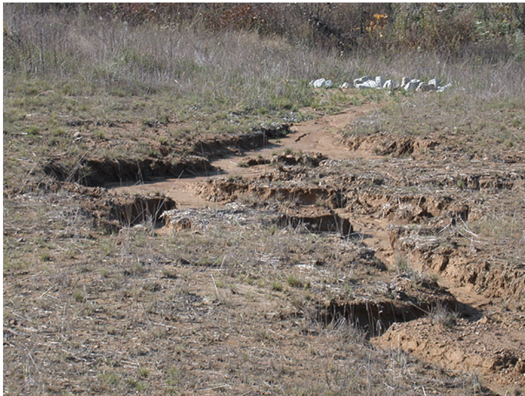
Figure 3. A) Aquatic sampling site #1, note the abundance of downed timber. The sampling reach extends a short distance into the adjacent forested area. B) Erosional washout near aquatic sampling site #1 in the MPTR, Camp Atterbury, Indiana. Riprap in background has been placed, apparently, to control erosion. Photographs by Steve Taylor, 3 November 2003.
