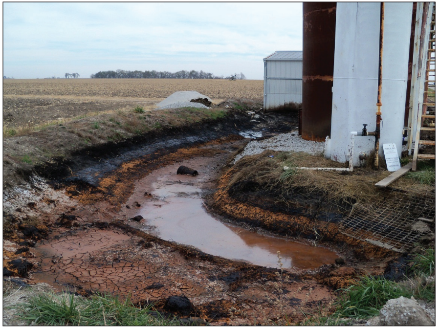
Figure 15 Aboveground storage tanks with discolored soil and water. Photograph by Matt Villicana.
