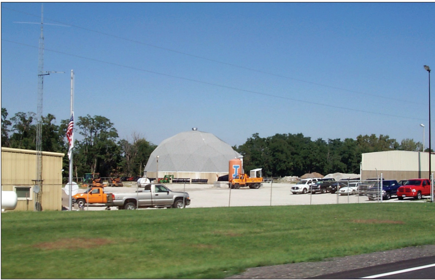
Figure 18 IDOT maintenance facility. Photograph by Greg A. Kientop.
